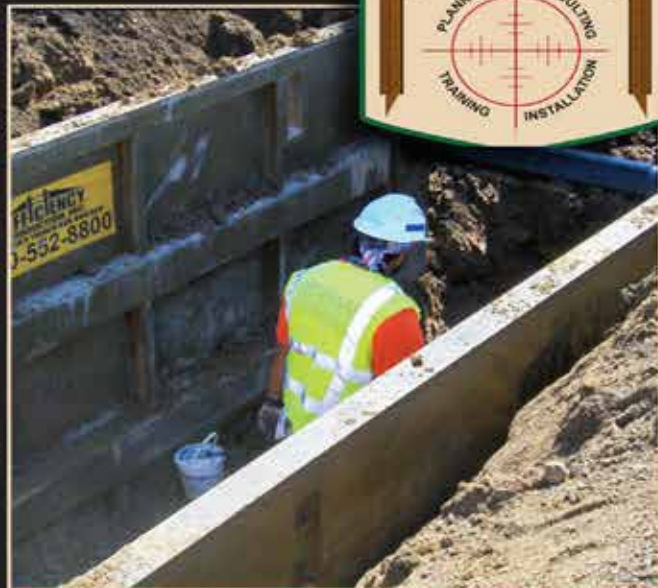
Steel Trench Box
