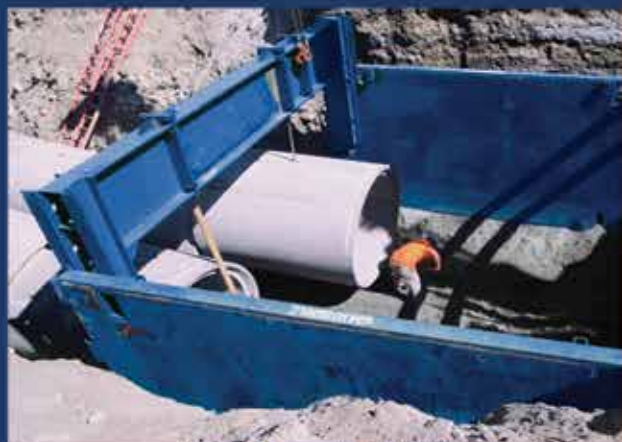
Steel Trench Shields
