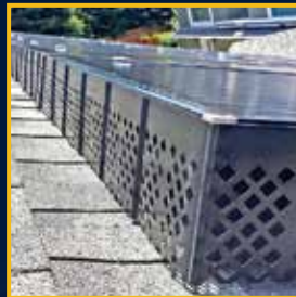
Solar Panel Bird, Animal & Debris Protection
