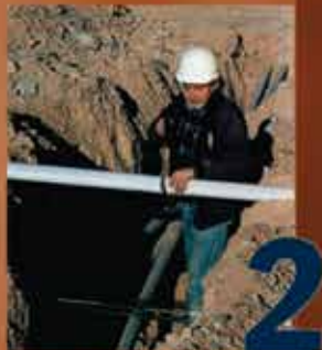
Step 2: Cut Split Duct Conduit to Fit
