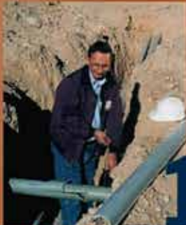
1 Step 1: Remove Damaged Conduit
