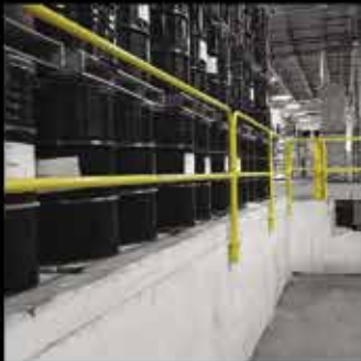
SHIPPING PIT RAILINGS
