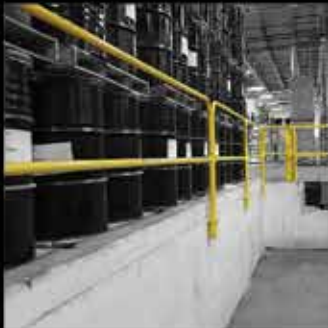
SHIPPING PIT RAILINGS
