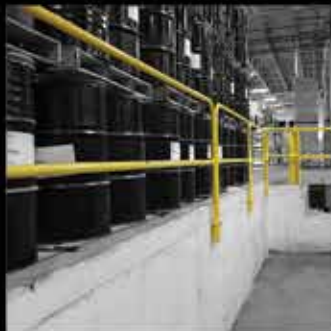
SHIPPING PIT RAILINGS
