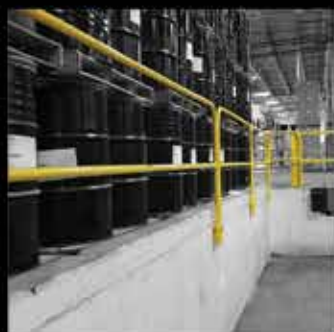
SHIPPING PIT RAILINGS
