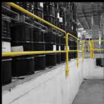
SHIPPING PIT RAILINGS
