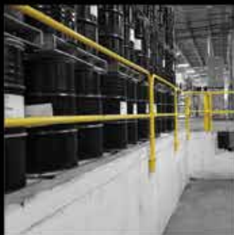
SHIPPING PIT RAILINGS
