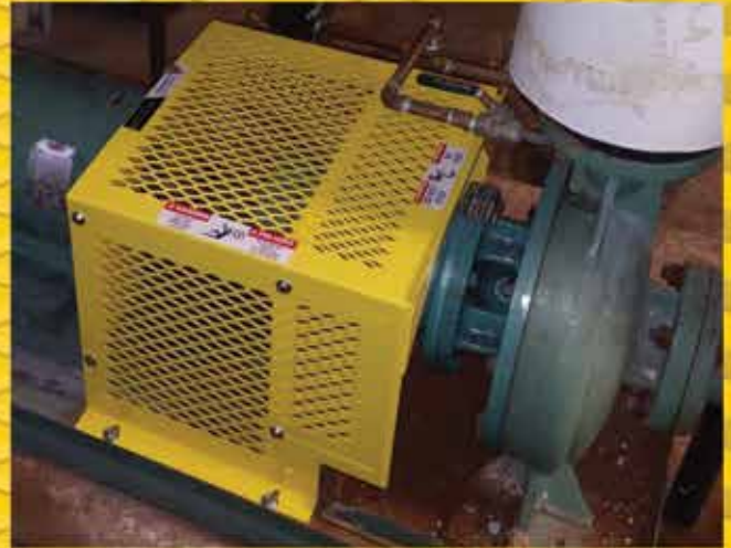
Sliding Panel Open for Packing Gland Adjustment
