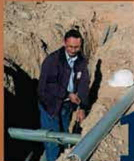
1 Step 1: Remove Damaged Conduit
