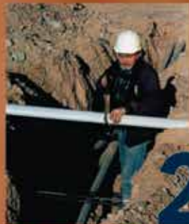
2 Step 2: Cut Split Duct Conduit to Fit
