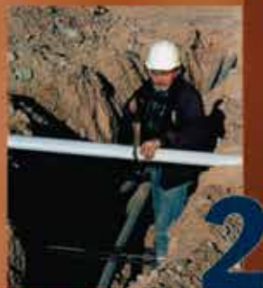
2 Step 2: Cut Split Duct Conduit to Fit
