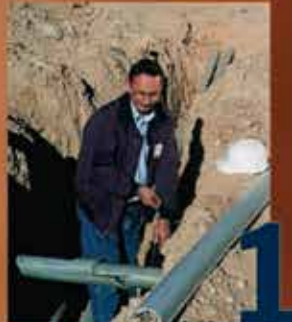
1 Step 1: Remove Damaged Conduit
