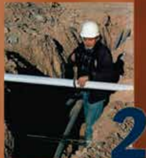
Step 2: Cut Split Duct Conduit to Fit
