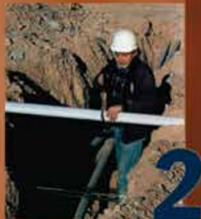
Step 2: Cut Split Duct Conduit to Fit
