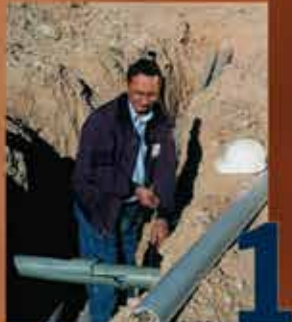
Step 1: Remove Damaged Conduit
