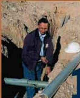
1 Step 1: Remove Damaged Conduit
